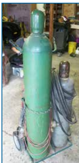
Oxy-Acetylene tanks and cutting rig owned not rented
